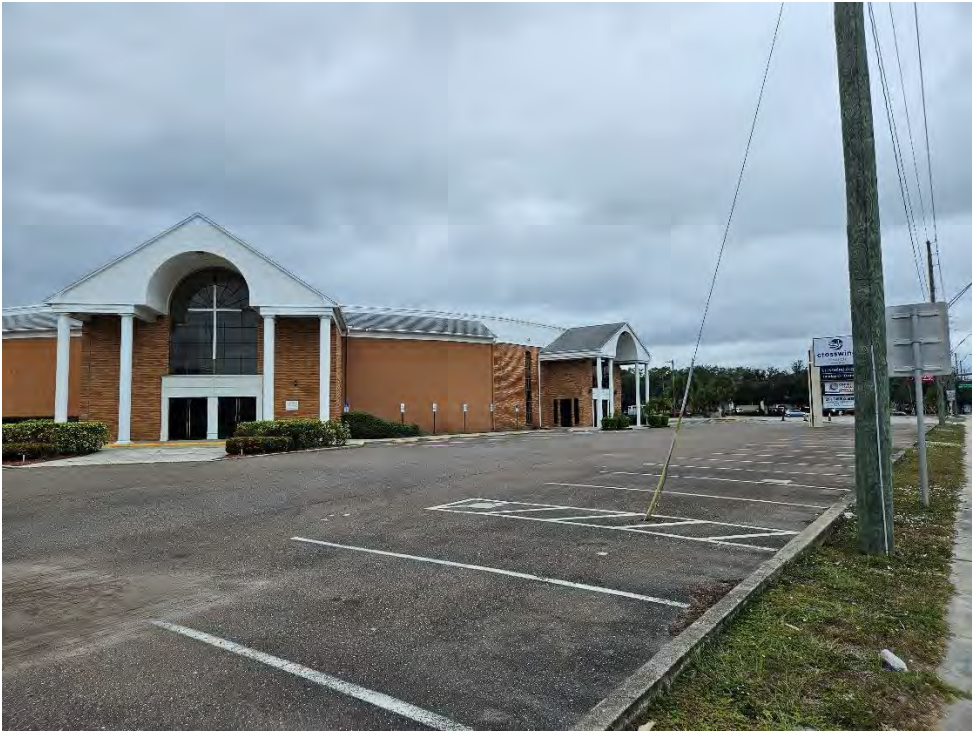
Looking at the subject site
